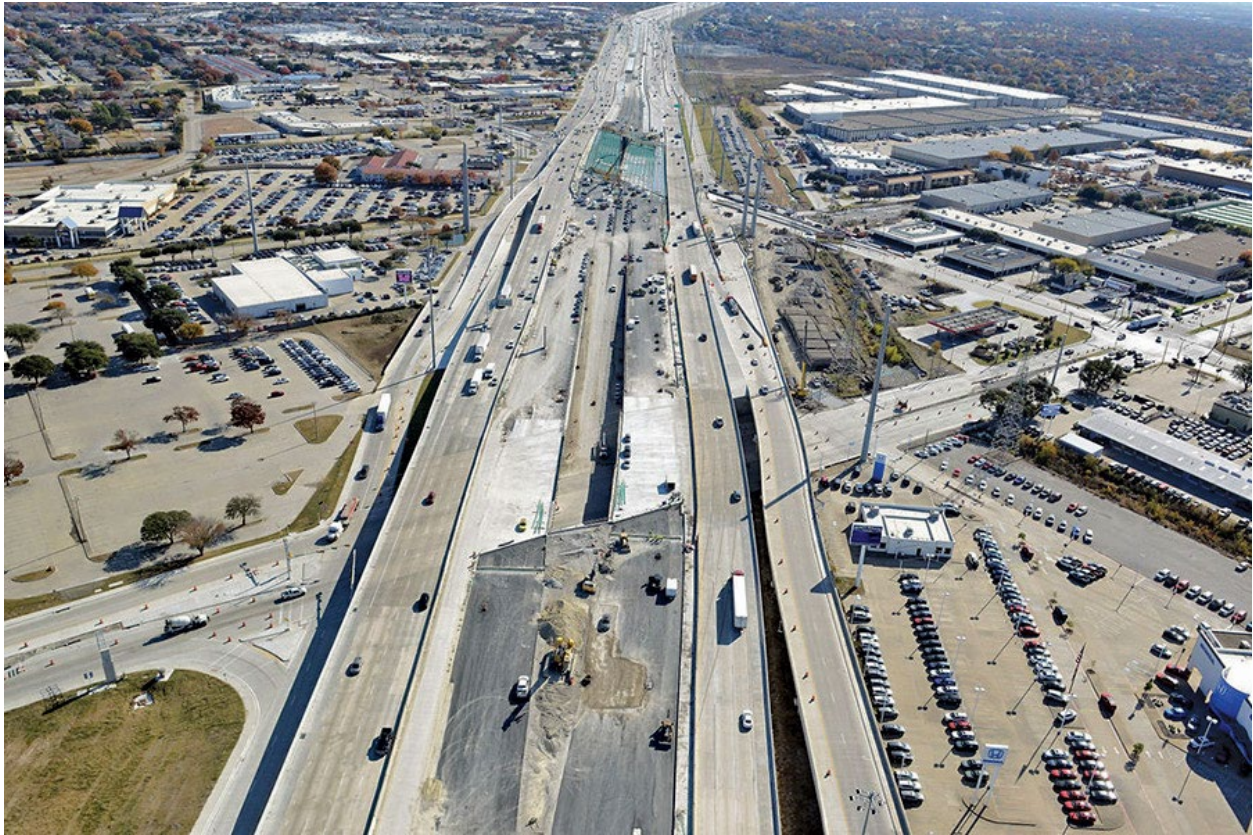
The $1.6B LBJ East project, scheduled for completion next year, is a testament to Morris' consensus-building approach. Photo courtesy Pegasus Link Constructors
